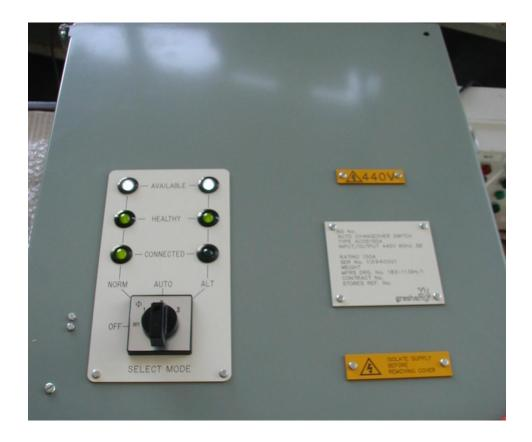
The Automatic changeover switch (ACOS) provide the capability to automatically switch a load between a 'Normal' and an 'Alternative' supply. Switching employs mechanically interlocked contactors and is controlled by electronic monitoring of the supply. Override facilities are provided which allow for manual selection of either power source.
