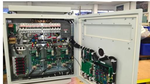
The chargers consist of an input automatic changeover switch, an auto transformer, rectifier modules, and output distribution.
