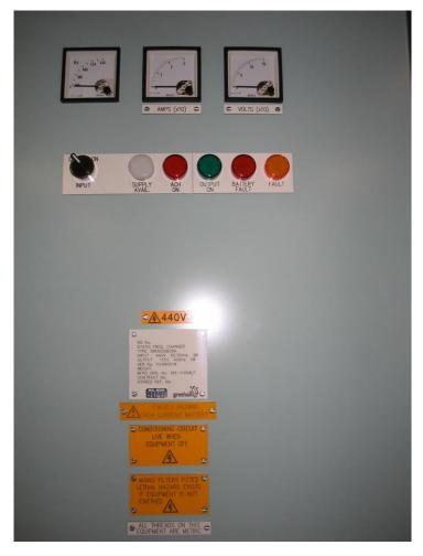
The 1BR3000B30A Static Frequency Converter (SFC) provides a high quality output of 115v 400hz 1 $\varphi$ @ 3000VA from an input of 440v 50/60hz. The integral valve regulated lead acid battery will support the output for 30 minutes in the event of an input supply failure.
