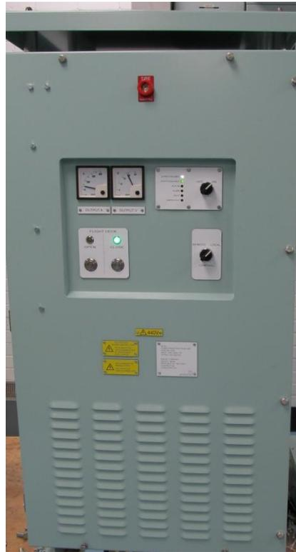
The Transformer Rectifier Unit 3RC15KE is intended for shipboard Helicopter Start applications. There are three basic modes of operation
