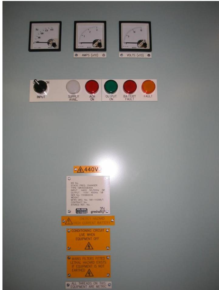
The 1BR3000B30A Static Frequency Converter (SFC) provides a high quality output of 115v 400hz 1 $\phi$  @ 3000VA from an input of 440v 50/60hz. The integral valve regulated lead acid battery will support the output for 30 minutes in the event of an input supply failure.
