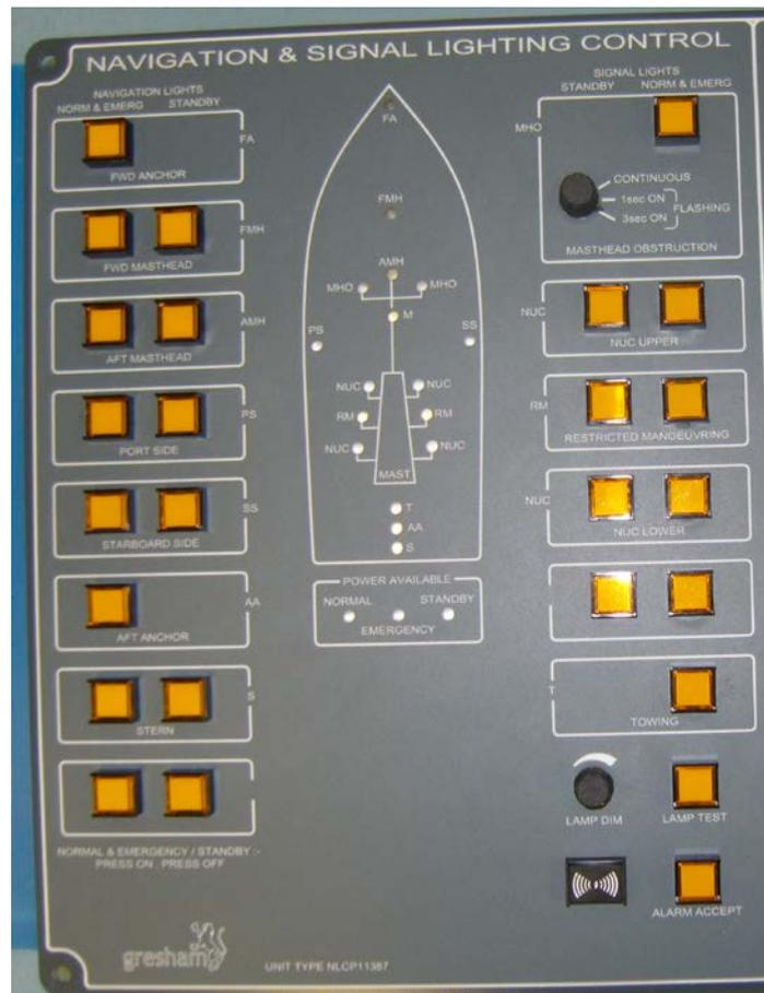
The navigation and signal lights are controlled from a panel that fits into a console located on the bridge. This is linked to a power panel located within the console.
