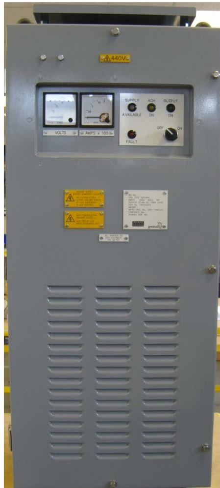
The Transformer Rectifier Unit type 3RC5kA provides a high quality output of 27.4 volts dc.
